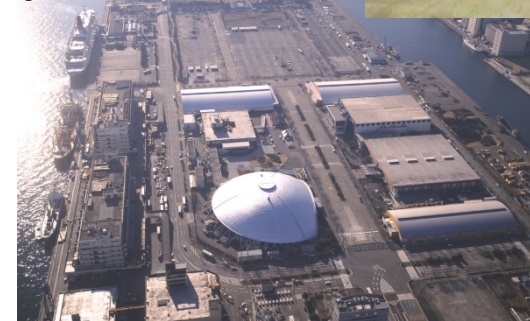
Bird's eye view of Harumi Convention facilities.
